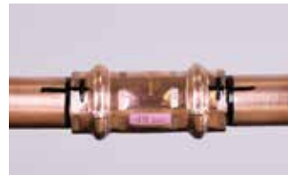
3. Mark the completed joint
