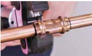
1. Align jaws squarely on the fitting
