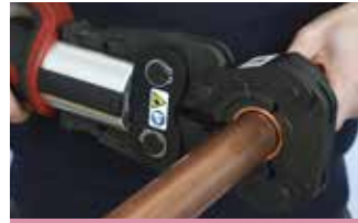
3. Complete the joint with the press tool
