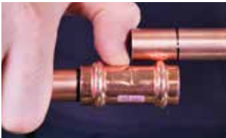
7B. Check the depth mark
